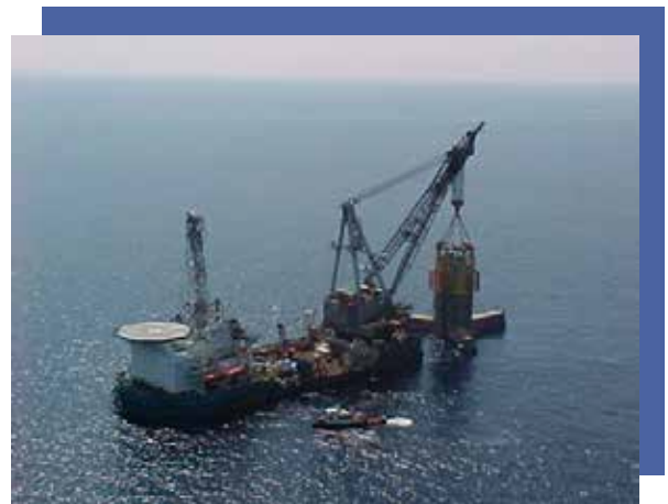
Installation of a Seastar® submersible hull.
